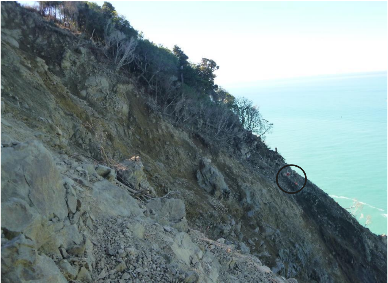
Figure 1: Rope access technicians (circled) scaling head scarp, Slip 7 north of Ohau Point, Kaikōura, Feb. 2017. Photo: R.Musgrave
