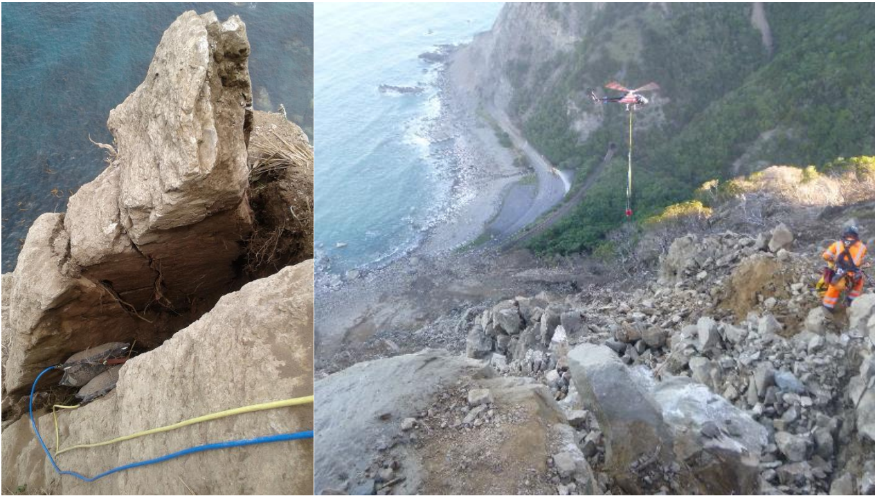
Figure 4 (left): Air bags used to remove an unstable column of rock while operators retreat to a safer location, Slip 10, south of Kaikōura. Photo R. Musgrave. Figure 5 (right): Sluicing to remove loose debris below abseiler, Slip 7, north of Ohau Point, Kaikōura. Photo R. Musgrave
